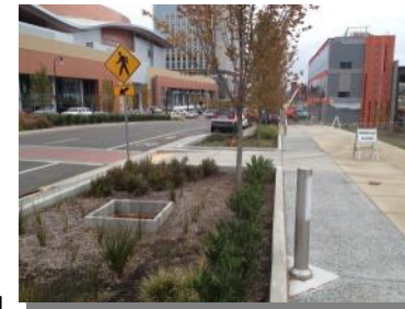
An example of more modern storm water collection practices which would reduce and/or eliminate stormwater discharge into the nearby Payette River
