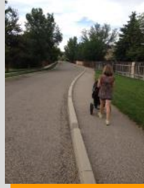
Extruded Curb Side-walks
