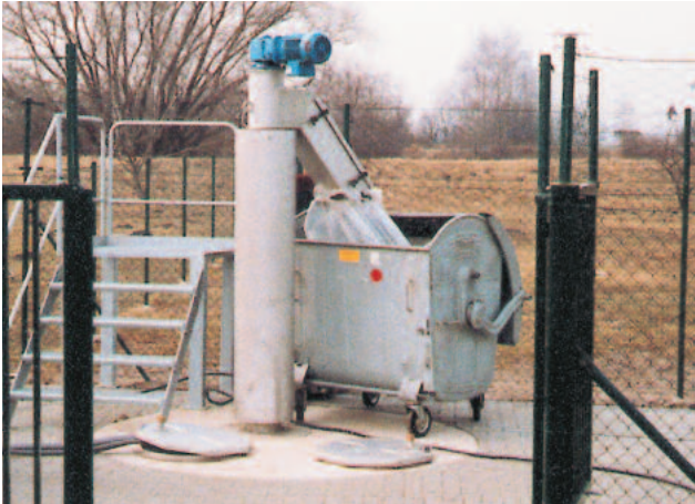
Thermally insulated and heat-traced unit
