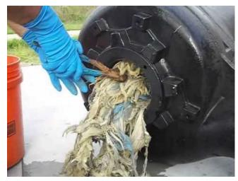
Non-flush items like masks, cleaning cloths, wipes and diapers cause wear and tear to a lift station pump and are time consuming to remove. KEEP COSTS DOWN, don't flush disposables, only toilet paper.
