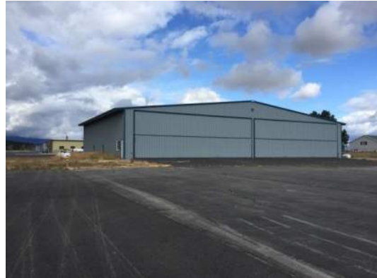
Box Hangar - U70 Source: T-O Engineers
