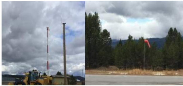
U70 Rotating Beacon (Left) and Windcone (Right) Source: T-O Engineers
