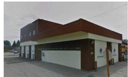
Fire Station Cascade, ID Source: Google Earth 2016
